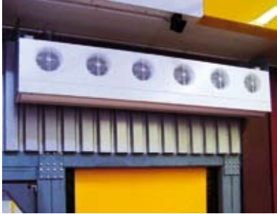
An INDUVENT device Type S. Horizontal installation above the door, the air intake section at the front.
