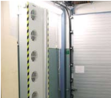
The vertical Type U with a sideways air intake section.
