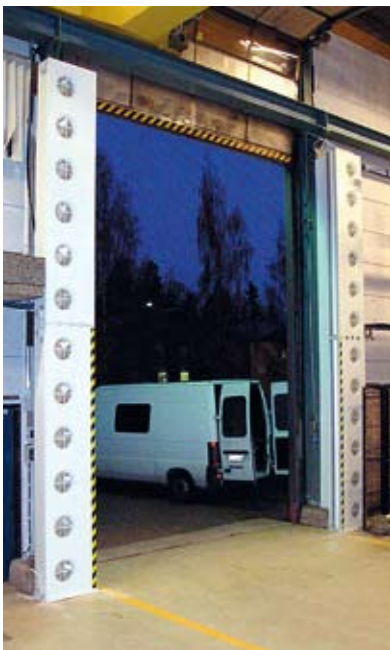
The vertical S dual system with its air intake section at the front effectively shields this very high door area.
