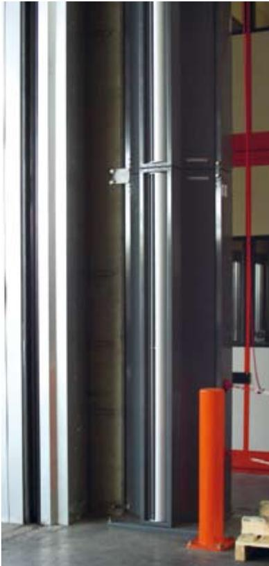
A RATIOVENT system vertically installed with two devices one over the other. The patented EVOLVENT® nozzle saves up to 40% energy compared with systems with conventional lamella technology.
