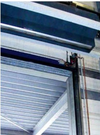
Also horizontally installed above the door, the EVOLVENT® nozzle provides for an optimal screening performance down at ground level.
